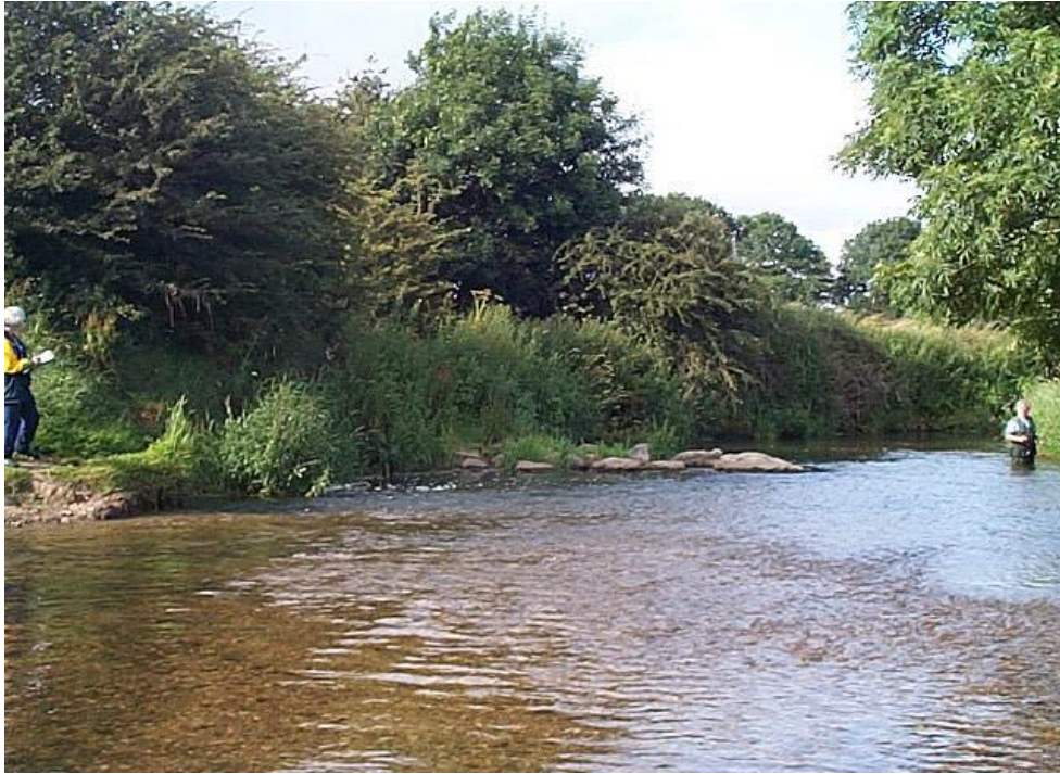
Plate 5. Restoration method on the Malmesbury Avon, using large Sarsen stones to create current deflectors and gravel to create a riffle.
